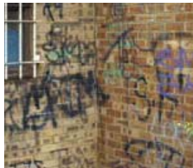
Cleaning the graffiti
